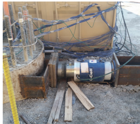
Lateral load test setup
