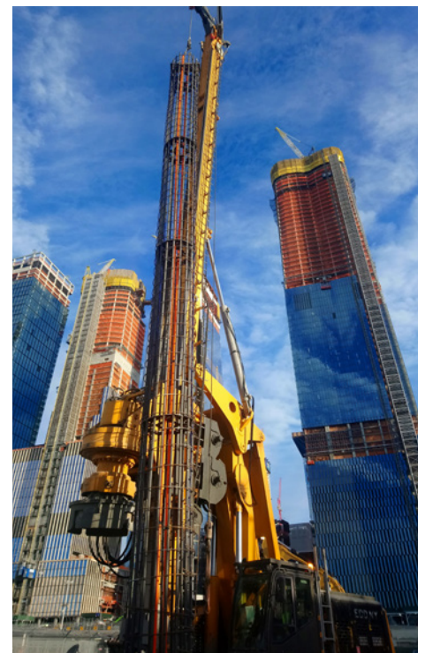
Installing the O-Cell assembly
